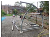
Photo of existing cycle shelter to be refurbished
