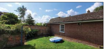
Photo of current wall prior to re-building of collapsed area
