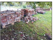
Photo of salvaged bricks from collapsed wall cleaned and ready to be used to rebuild the wall.
