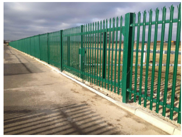
2.4m High Paillisade Fence
