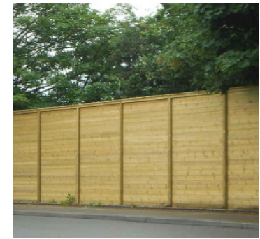
4m High Acoustic Fence
