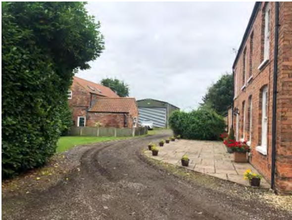
Image .01 – View of the application site looking South West.
