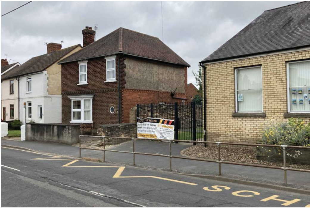
B. Existing Streetscape View
