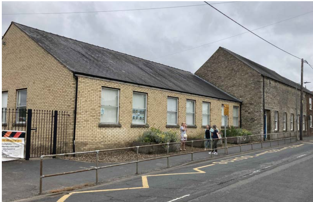
A. Existing Streetscape View
