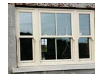
Windows - upvc cream mock sash
